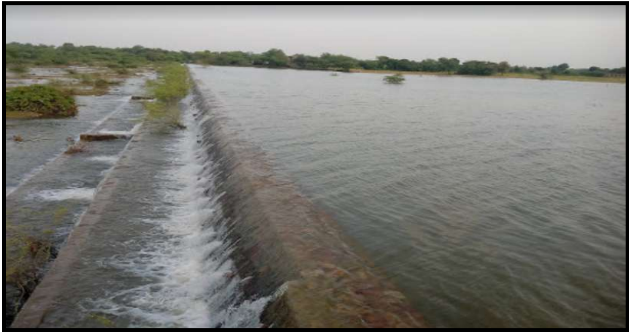
Figure: 01 Photograph of Ummedsagar dam Shahpura (Bhilwara) during monsoon
